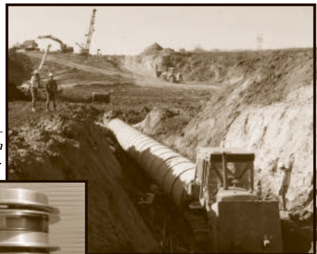
Job site view of a large-bore concrete pipeline in an open trench installation.
