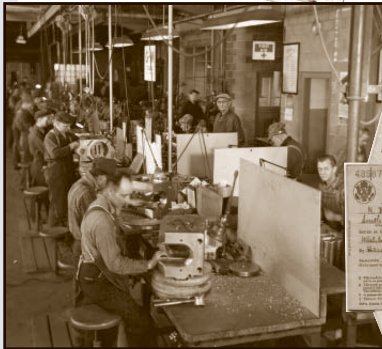
Besser Company employees working on the breech mount for 3" naval deck gun built during WWII.
